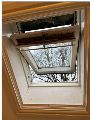
Photo - 14 Bathroom Velux rooflight.
