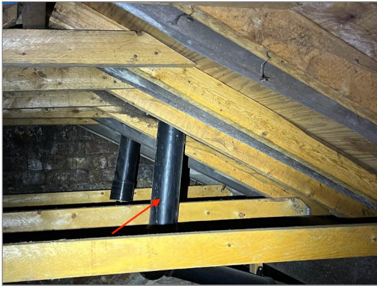
Photo - 37 Soil vent pipe visible in loft.
