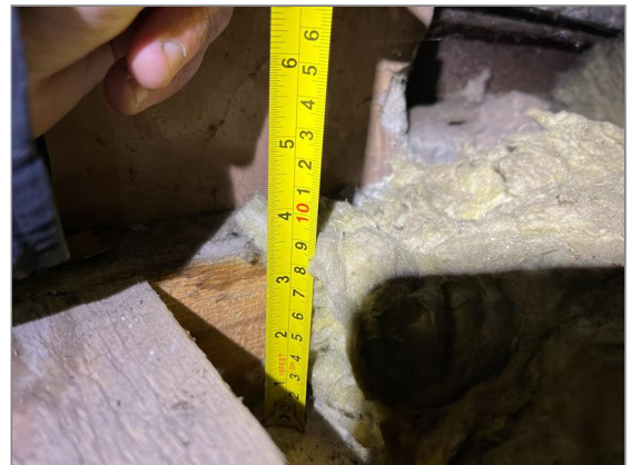
Photo - 25 Rear addition / utility room loft insulation - approx 90mm.
