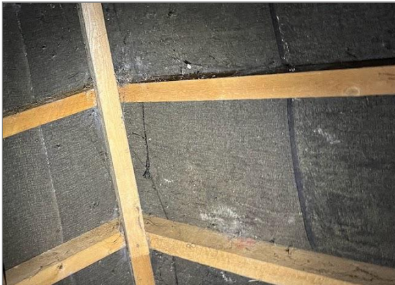
Photo - 3 Rear addition / utility room secondary waterproof layer (roofing felt).
