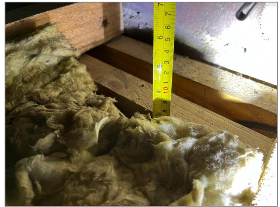
Photo - 23 Loft insulation (main loft) - approx 80mm
