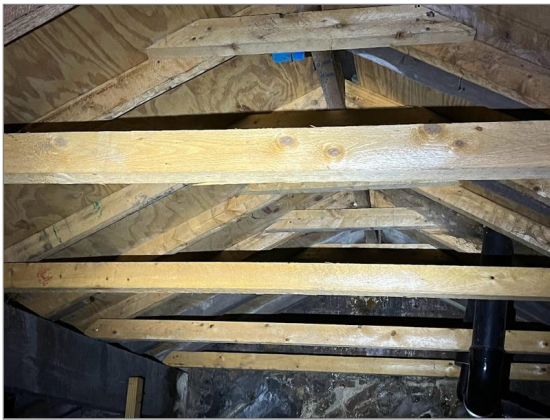
Photo - 16 Roof structure - replacement timbers.
