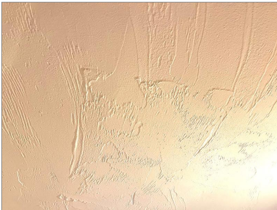
Photo - 26 Textured ceiling coating.
