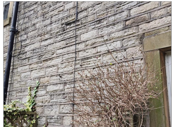
Photo - 13 Walls structurally sound and in fair condition for age
