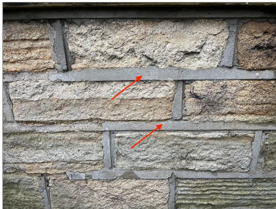
Photo - 12 Cement based mortar pointing.
